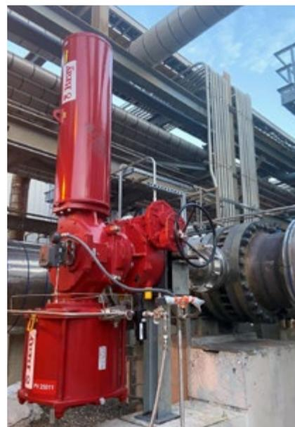
**Tri Lok triple offset butterfly valve installed with Series 98 Scotch yoke pneumatic actuator and digital positioner. The two valve packages have greatly increased operational efficiency in the propane dehydrogenation process.**
