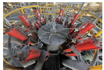
After 6 months of operation, these Bray Series 768 Knife Gate Valves required no service, and returned to continuous duty.
