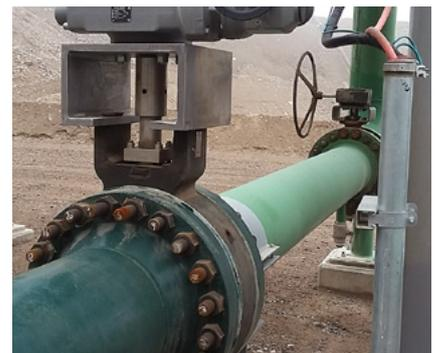
*The McCannalok metal-seated double offset butterfly valve has provided more than five years of continuous service, with no failures and no maintenance required.*
