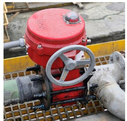
*Bray Series 39L ceramic lined control valve with Series 70 electric actuator provided improved control precision with increased operational lifespan.*
