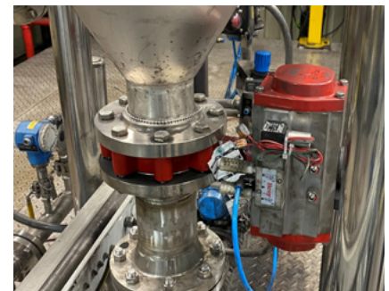
The Bray automated valve package (above and below) performed with impressive results, and has now replaced more than 20 pinch valve assemblies.
