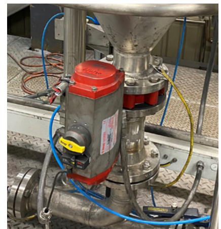
The Bray automated valve package (above and below) performed with impressive results, and has now replaced more than 20 pinch valve assemblies.
