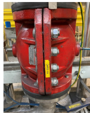
Existing pinch valve with EPDM sleeves that were tearing frequently.
