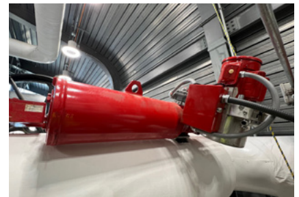
Scotch yoke failsafe actuator with integrally mounted hydraulic power unit, installed in steam application.
