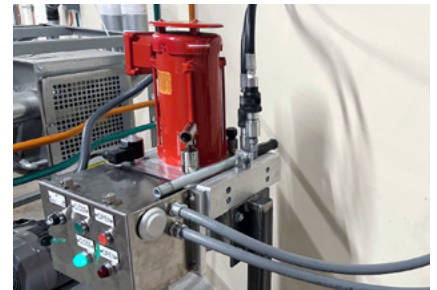
Upper image shows valve and actuator mounted in very tight space. Lower image shows the actuator's hydraulic power unit mounted remotely, due to the space constraints near actuator.
