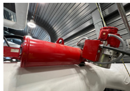
Scotch yoke failsafe actuator with integrally mounted hydraulic power unit, installed in steam application.
