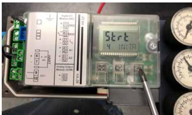
3.2.7 Upon successful completion of calibration, the status line will display “FINISH”. Press the Menu Button
